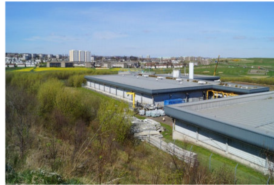
Nigg Waste Water Treatment Works
